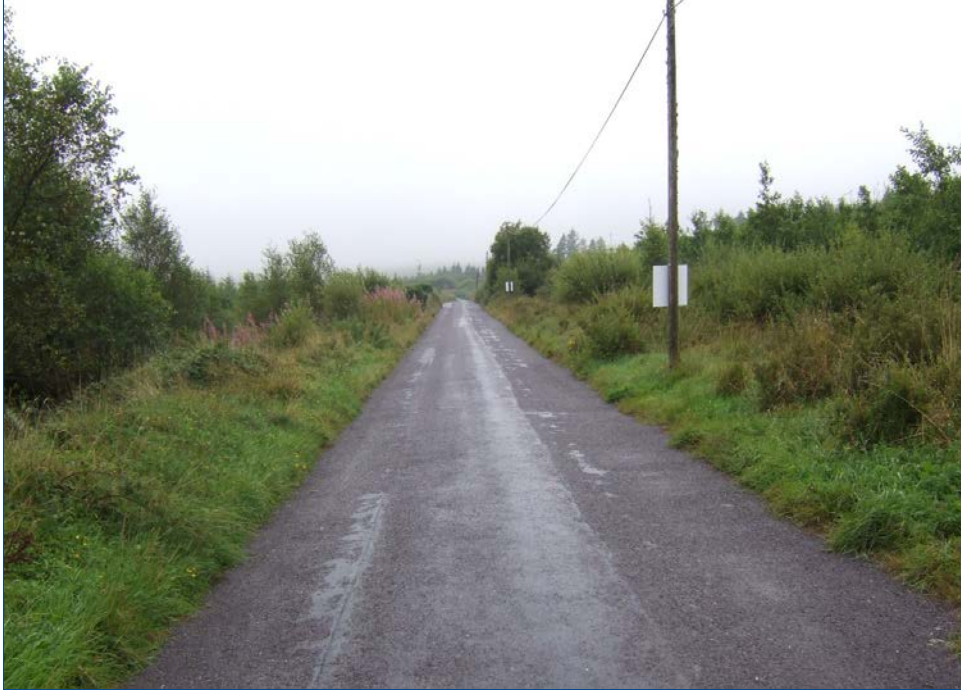
Plate 1. The cable will be laid almost entirely within existing roads and tracks (BL3). Roads are typically edged by grass verges (GS2). View is along road just south of Ballyvouskill substation, looking south-westwards.
